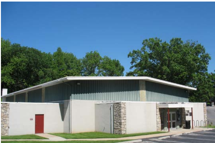
Existing Hughes Building
